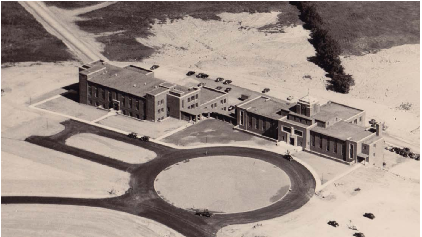
An aerial view of Le Moyne College during its construction.
