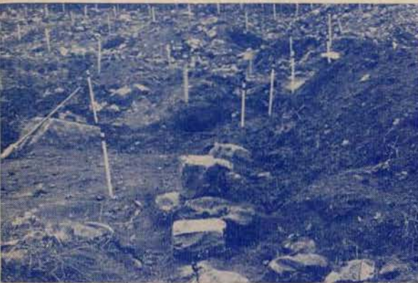
▼ Foundation stones of the Church, facing the St. Lawrence.
